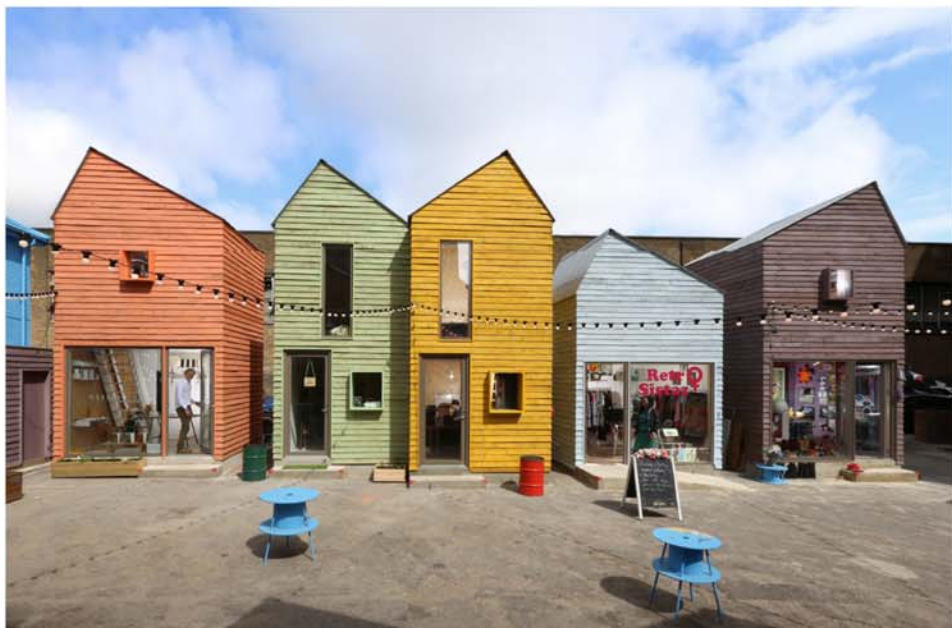
Photos Jan Kattein Architects, Warren Cooper
