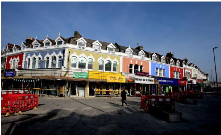
New shop fronts at Bakers Arms.
