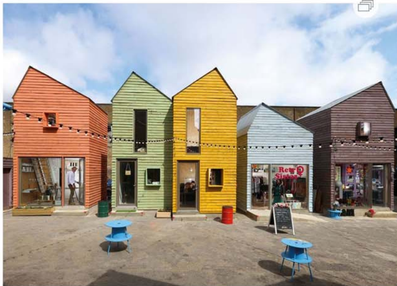
Turning the old car park into a 'place' for the short term, Jan Kattein Architects didn't redo the serviceable surfaces at the centre of Blue House Yard.
